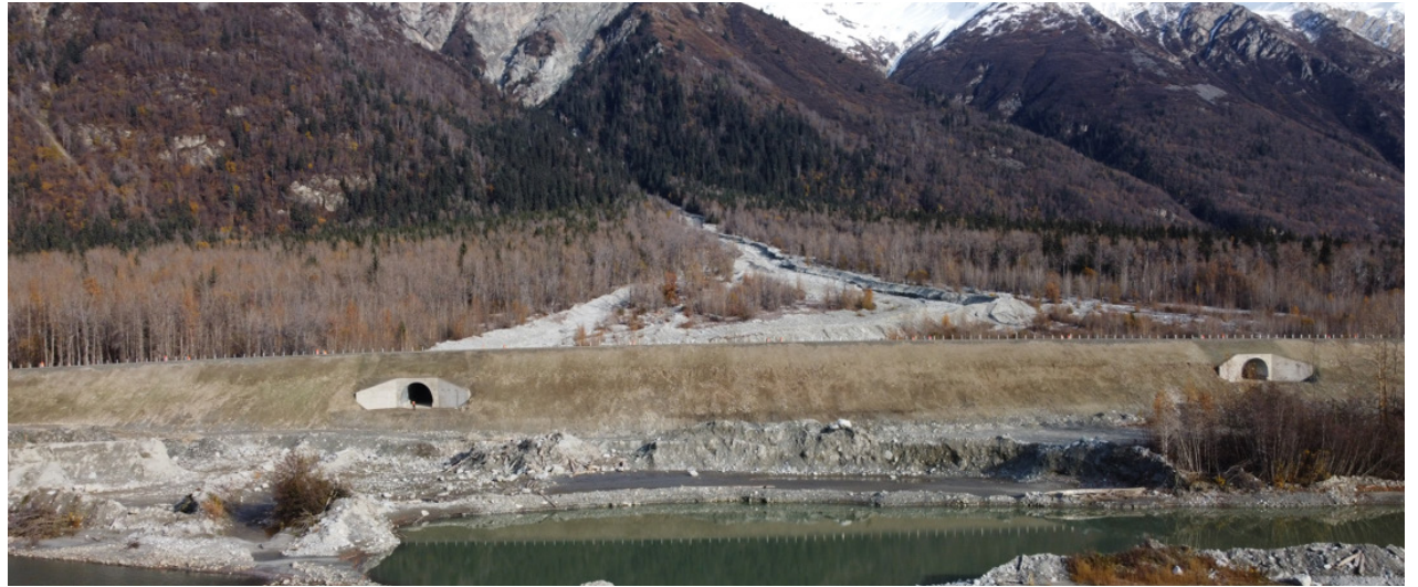
Figure G-8. Haines Highway MP19 project with elevated roadway.
