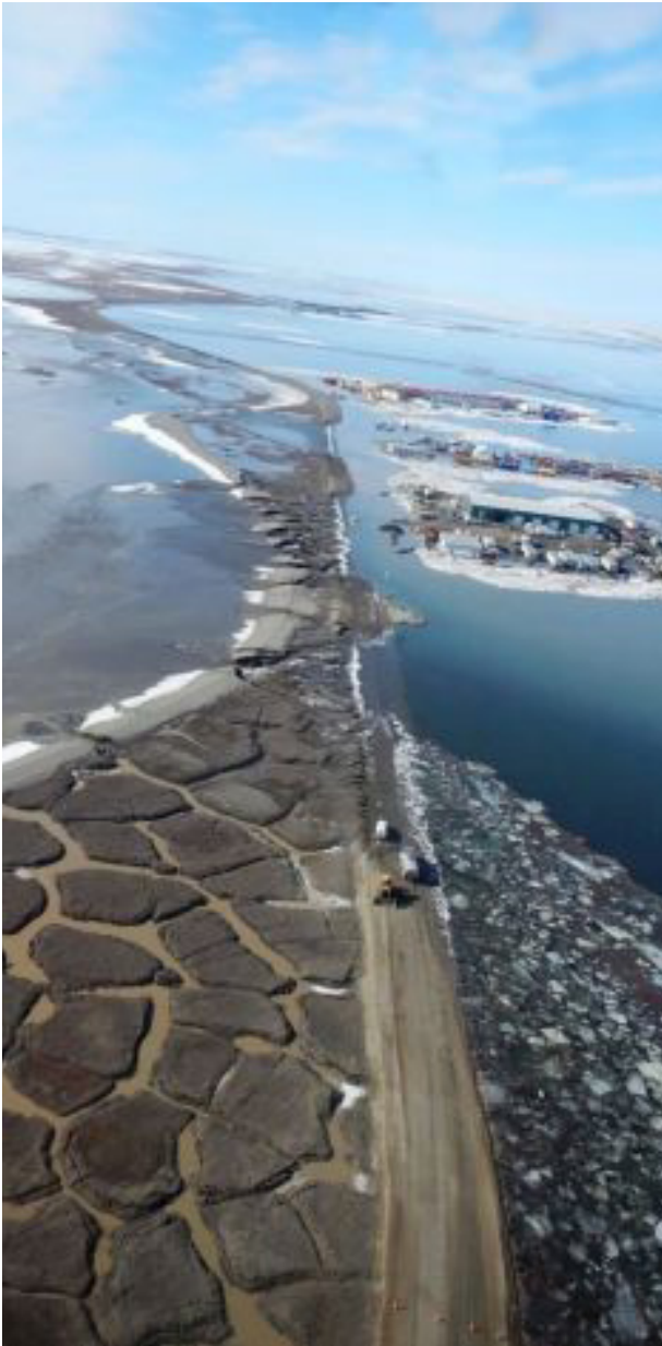
Figure G-7. Dalton Highway—2015 flooding.
