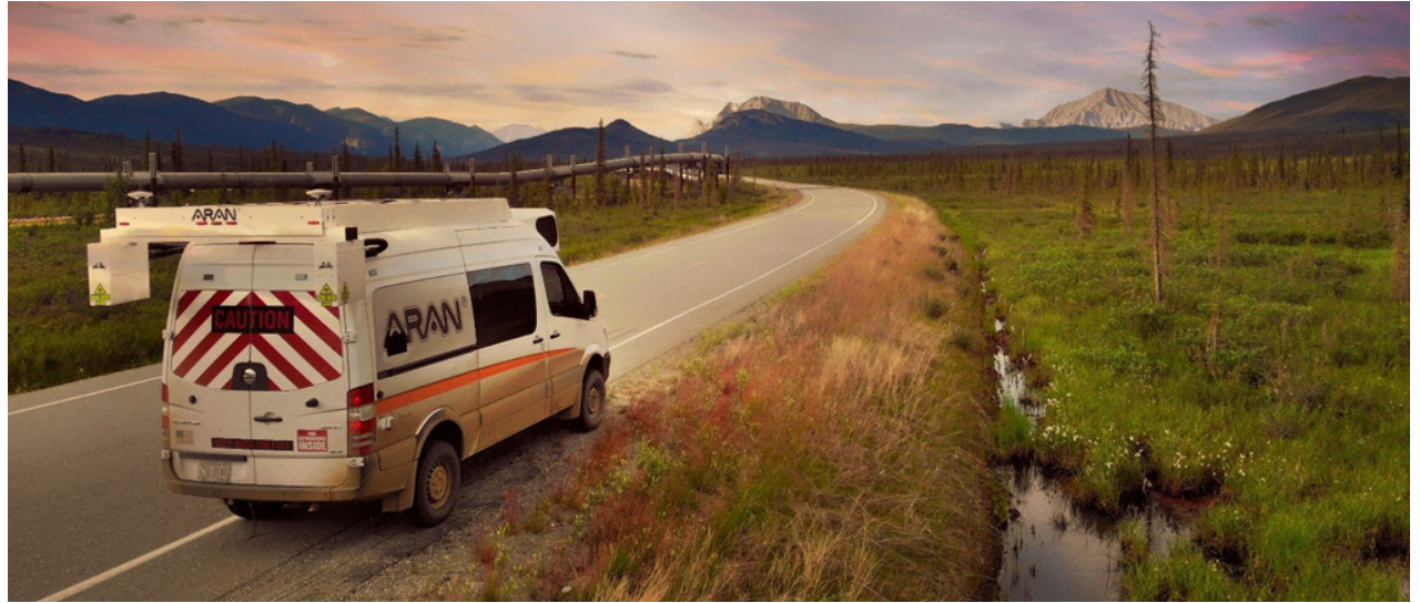
Figure C-1. Dalton highway stable embankment. Source: Fugro.
