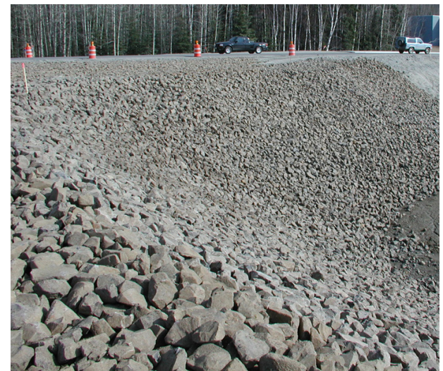
Figure G-5. ACE on Thompson Drive, Fairbanks
