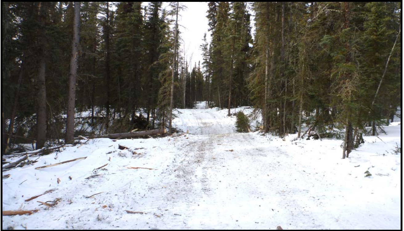
Figure 16: Proposed realignment near station 245+93. Photo is looking west at wooded hill area. Drilling in this area indicated frozen ice-poor sand or silt subsurface soil.
