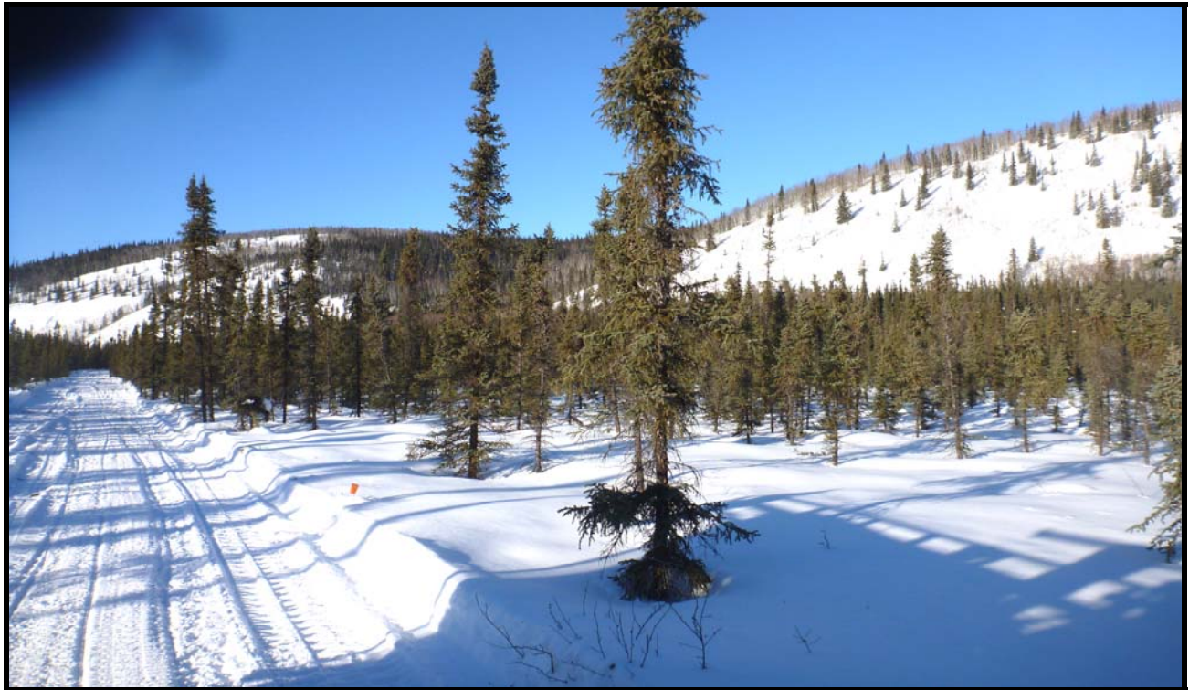
Figure 10: Proposed realignment near station 116+80. Photo is looking northwest at the alignment to the left of the photo and hills bounding the alignment to the north. Drilling indicated ice-rich subsurface soils in this area.
