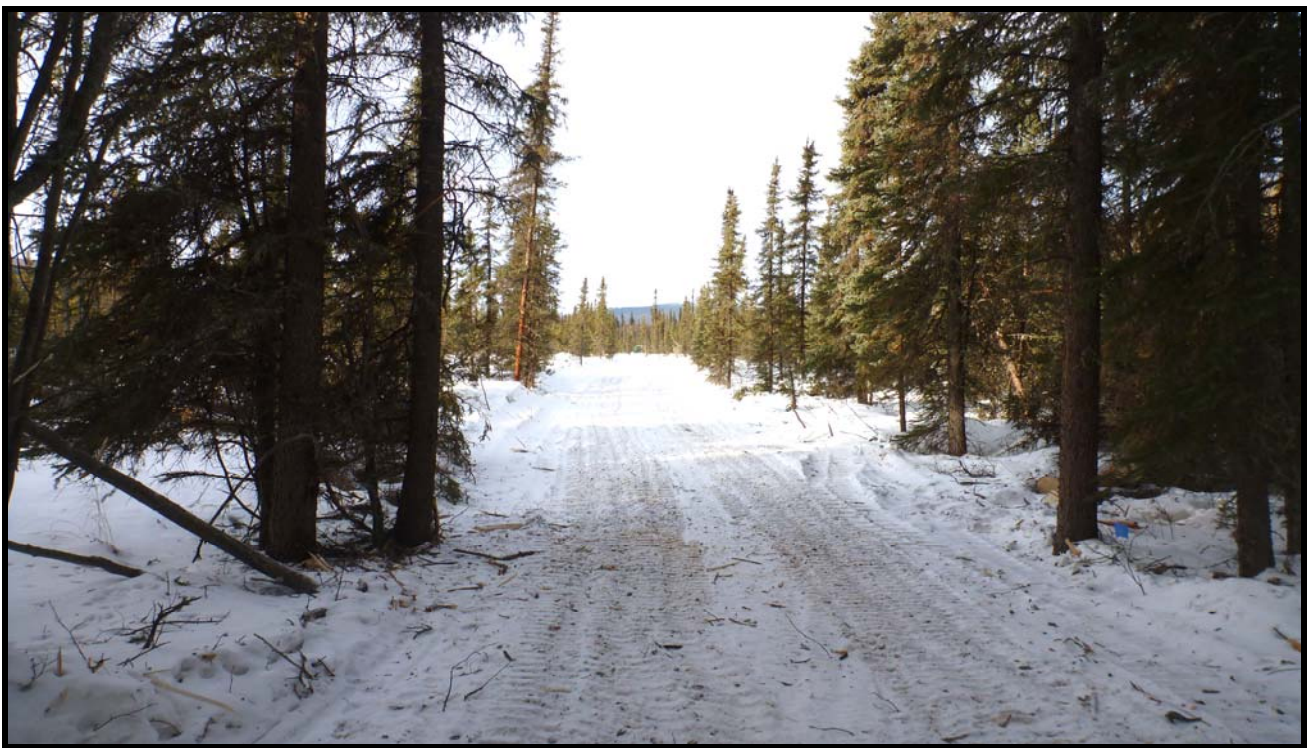
Figure 15: Proposed realignment near station 224+15. Photo is looking west at abrupt change from wooded hill slope area to flat low-lying open area. Drilling indicated wooded high ground areas generally consisted of ice-poor sand or silt, while flat low-lying open areas consisted of ice-rich soils.
