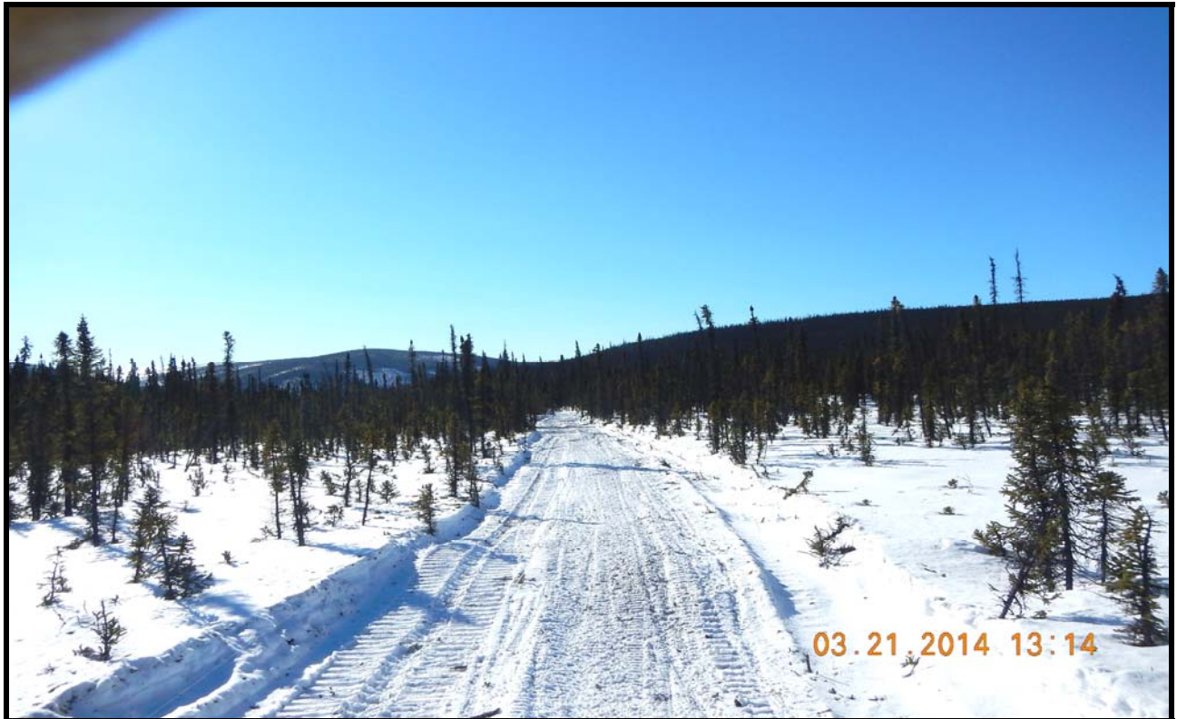
Figure 22: Proposed realignment near station 378+80. Photo is looking south. Drilling in this area indicated highly ice-rich subsurface silt soil.
