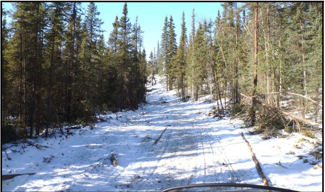
Figure 17: Proposed realignment near station 278+09. Photo is looking west at abrupt elevation change or bench located in the middle background. The change is also a transition between ice-rich and ice-poor surface soils.
