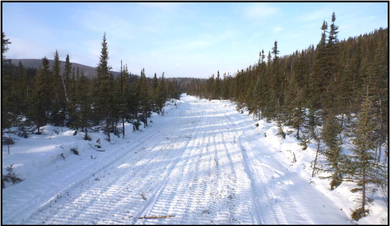
Figure 12: Proposed realignment near station 182+20. Photo is looking west. Drilling in this low lying area indicated ice-rich subsurface soils.
