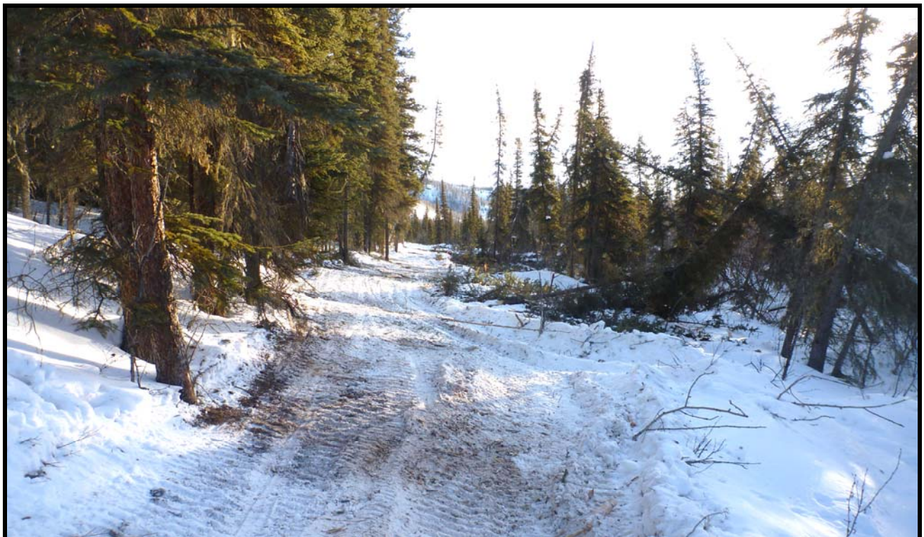
Figure 11: Proposed realignment near station 167+57. Photo is looking east with a hill slope to the left and low drainage area to the right. The hill slope could have unstable ice-rich silt material near the surface. Drilling indicated thawed soils underlying seasonally frozen soils in this area of the alignment.
